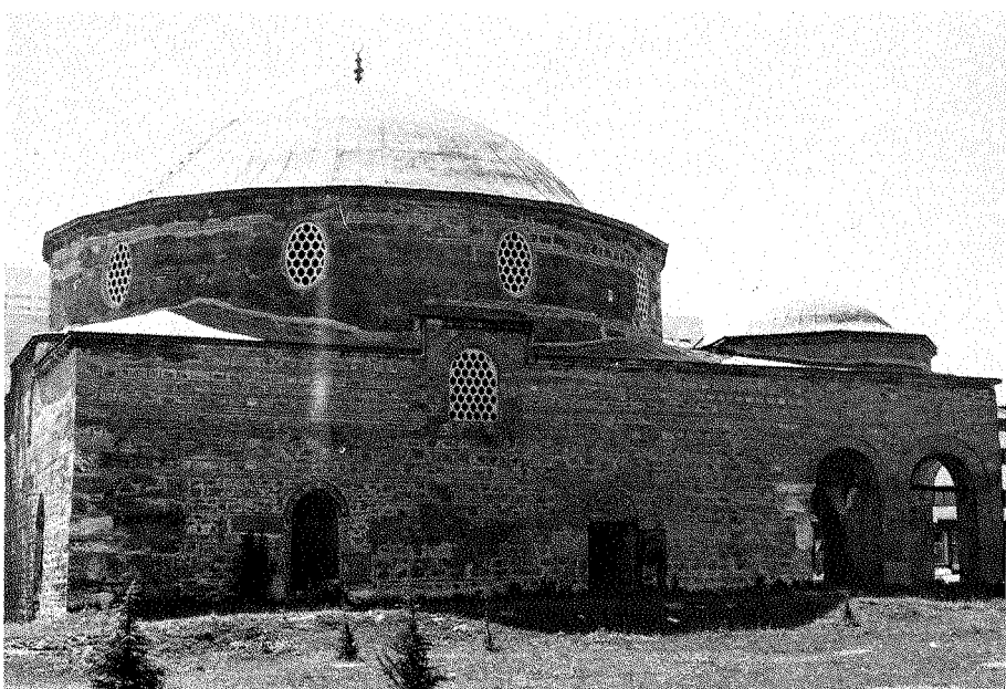
Fig. 7 — Stara Zagora, Hamza Bey Mosque in 1985 restoration almost completed
